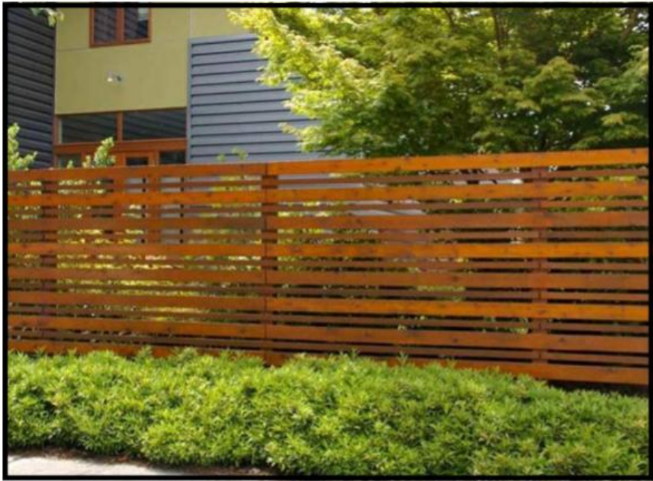
COURTYARD/PATIO RAIL/FENCE SPACING OF MEMBERS WILL VARY BASED ON APPROPRIATE PRIVACY MEASURES DICTATED BY SITUATION
