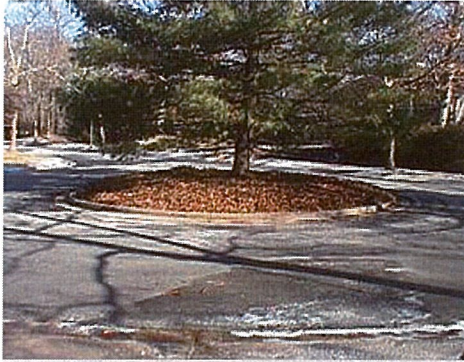
Rather than having a fully paved cul-de-sac bulb, site designers can incorporate pervious circles with vegetation that reduce the site's
